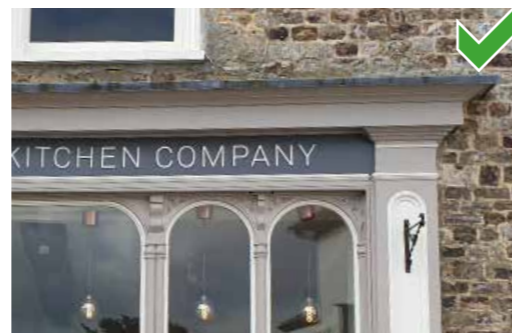
lead covered cornice providing protection for signage below.
